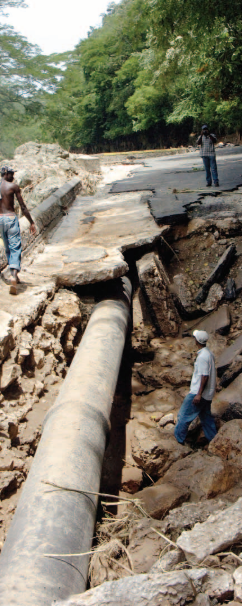
Damage inflicted by Hurricane Gustav on road in Bog Walk gorge
